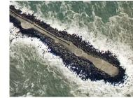
Breakwater is a barrier built out into a body of water to protect a coast or harbor from the force of waves. The idea is to
